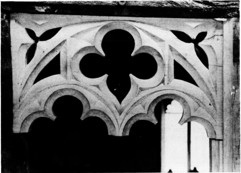
Fig. 13 Restored tracery for the second hall window
