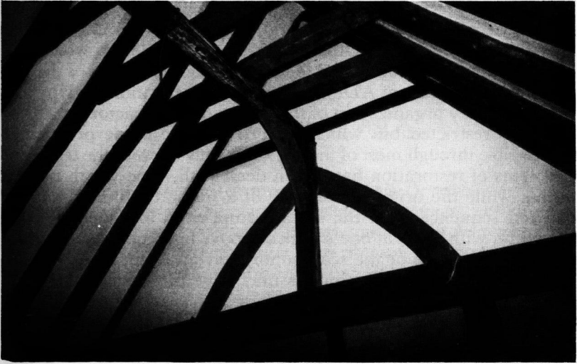
Fig. 16 Restored Truss I of the gallery
