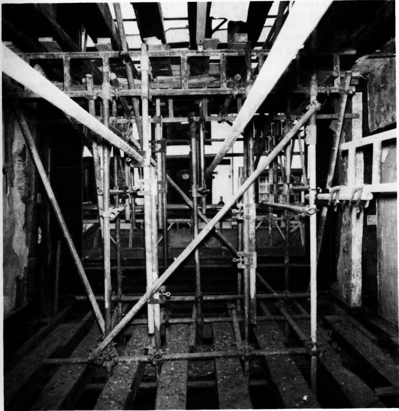
Fig. 8 Pre-contract scaffolding in 27 Cornmarket Street Photo: B.J. Harris Photographers, Oxford
